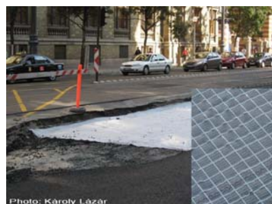
Figure 6. Knitted composite fabric used for driveway reinforcement
