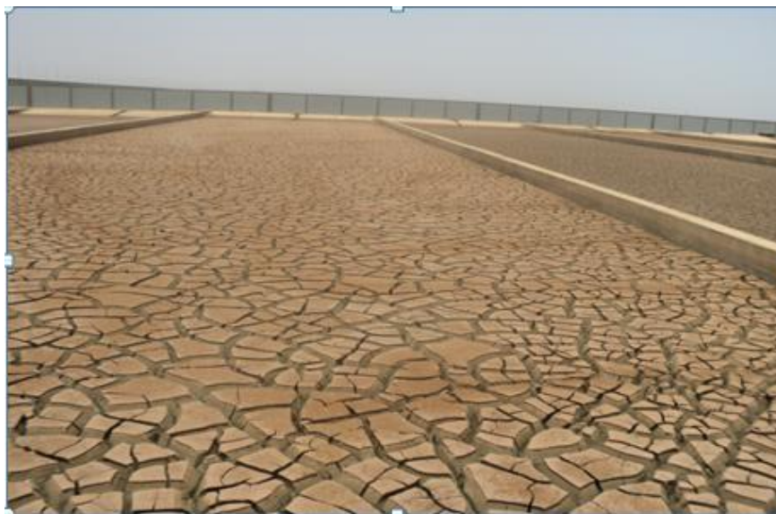
Plate 3: Drying of the sludge in large bonds
