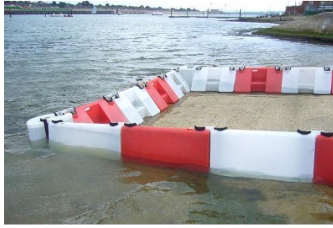
Figure 6. Example of plastic concave flood barriers [9]
