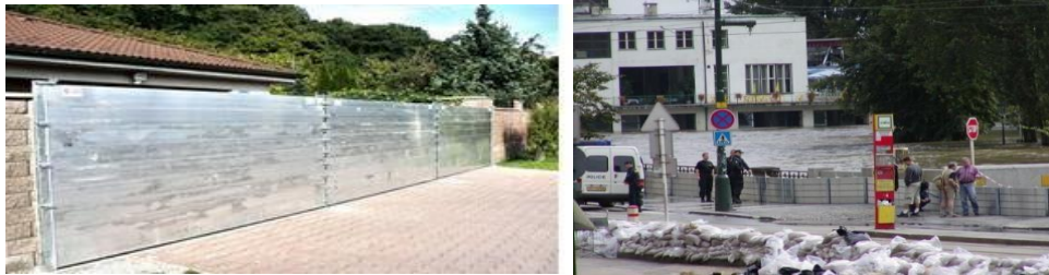
Figure 7. Examples of large metal systems of flood barriers
