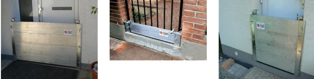
Figure 8. Examples of small metal systems of flood barriers – door protection [11]
