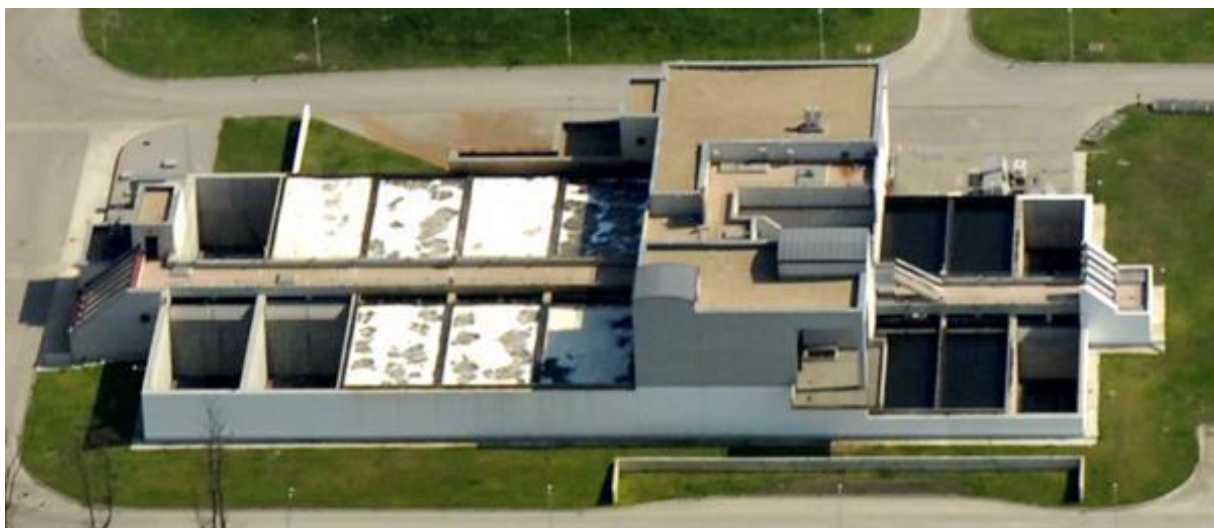
Figure 1. BIOFOR TM nitrification (left) and post-denitrification (right) biofilters – own picture
