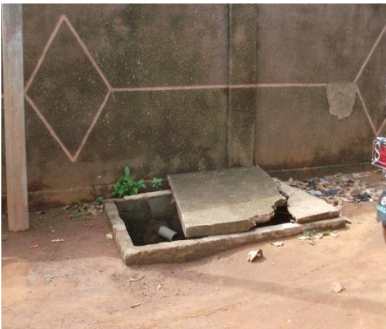
Photo 5: A functional sump but partially protected in district 1 of the town of Ouidah. Catch of sight Adoko E., June 2012
