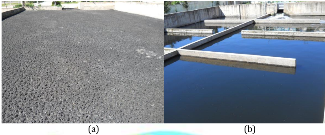
Figure 5: tertiary treatment, (a) sludge drying bed (pool chlorination)
