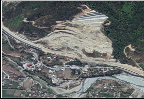
Figure 4 Actual situation (2018) of the slided area, Tr-El highway. [Source: Google earth]
